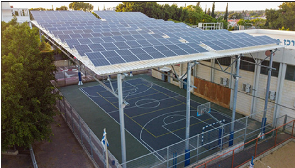
Image 1: Innovative use of sports ground for the production of solar-based electricity, providing a win-win solution with revenue for the municipality in Kfar Sava, Israel. Source: City of Kfar Sava
